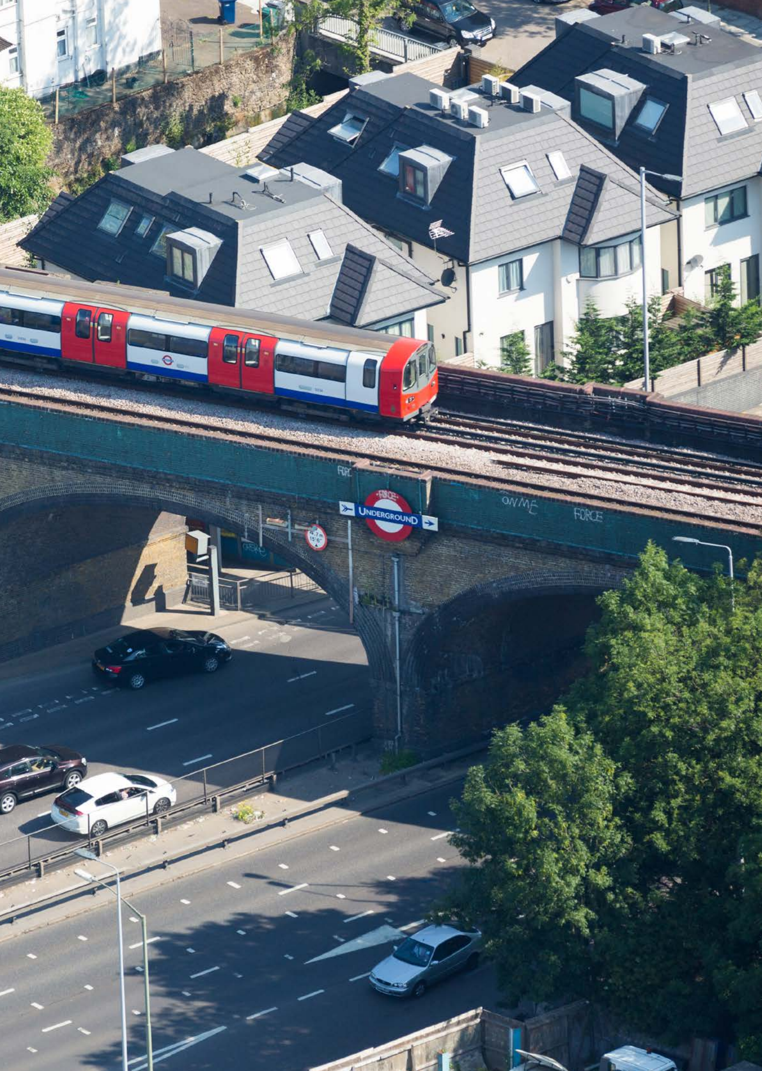
We have an extensive asset base that must be maintained
