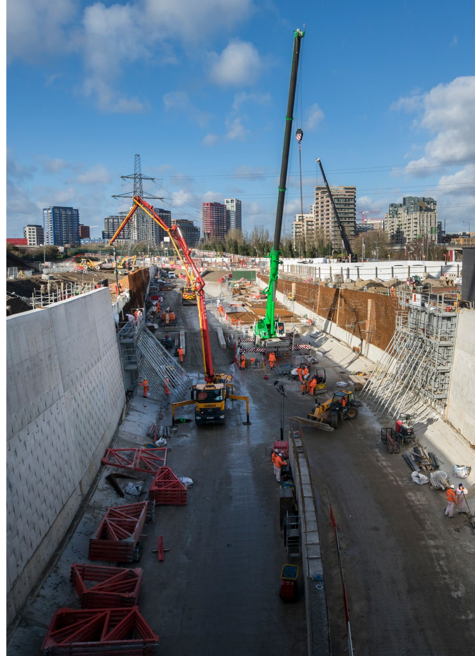
Work continues on the new Silvertown Tunnel, opening in 2025
