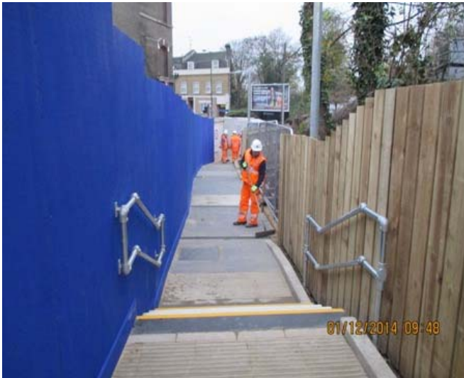
Temporary footpath at South Tottenham Station
