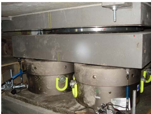
Temporary bearing and jacks required to lift the flyover
