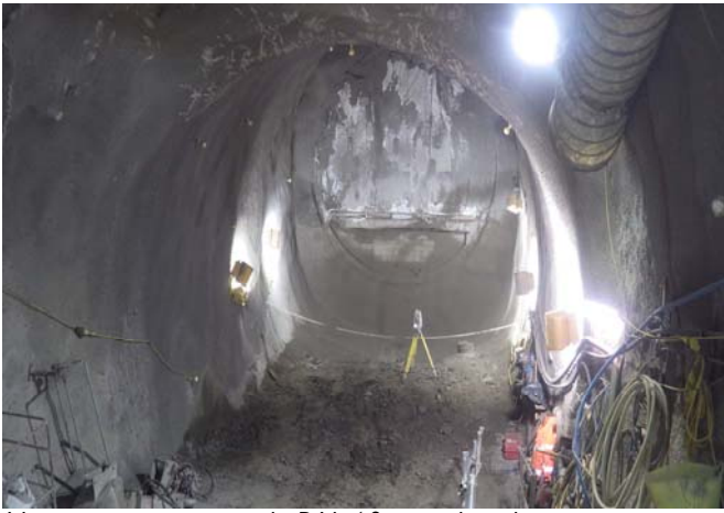
Victoria station upgrade PAL 10 completed
