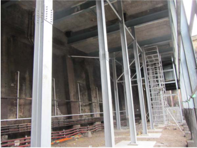
Floor strengthening steelwork as Farringdon
