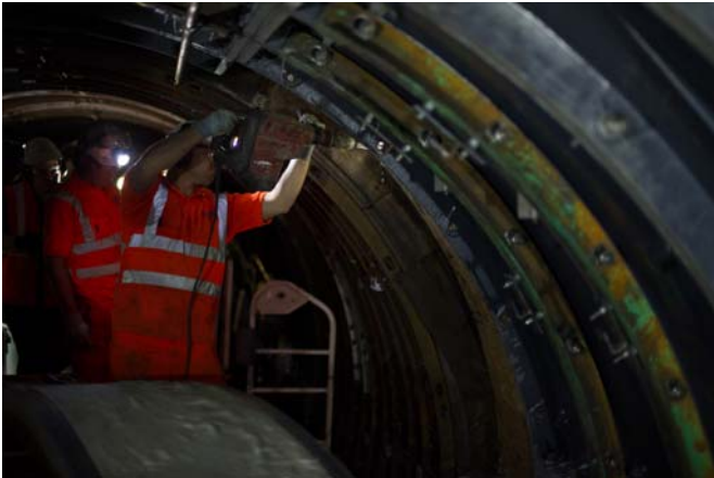
Baker Street to Bond Street tunnel lining works
