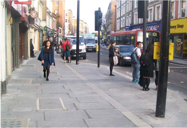
Earl's Court Road footway resurfacing
