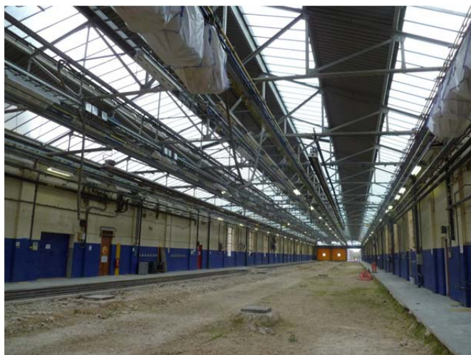
Ruislip depot shed prior to works commencing
