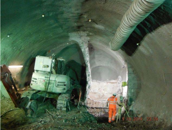
Bond Street sidewall drift for the new passageway
