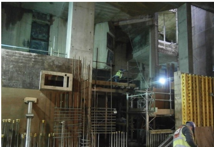
Fixing and pouring walls in the LU station box at Bank station
