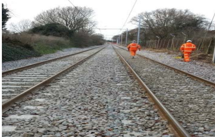
Twin tracking completed between Beddington Lane and Mitcham
