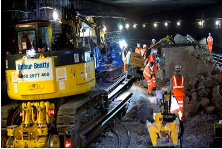
The train arrestor being removed at Tower Hill
