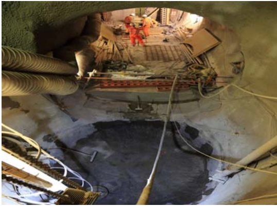
Bond Street lift shaft 3
