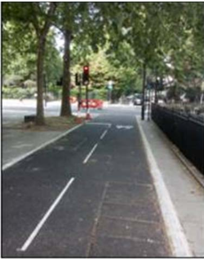
Grid Completed scheme at City Road / Colebrook Row (Islington)
