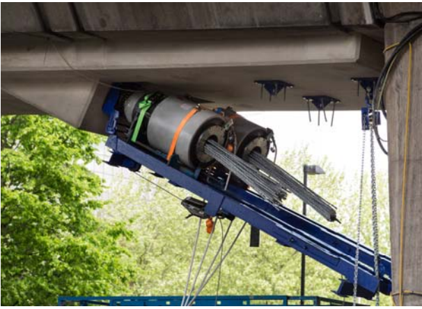
Tensioning of the internal long tendons
