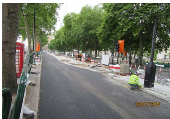
Victoria Embankment (East West route)
