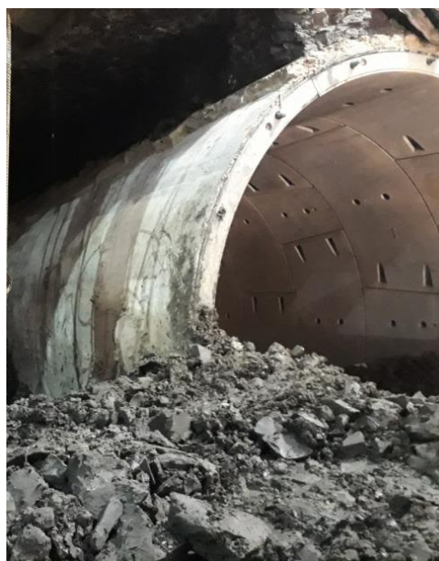
Demolition of the tunnel underway
