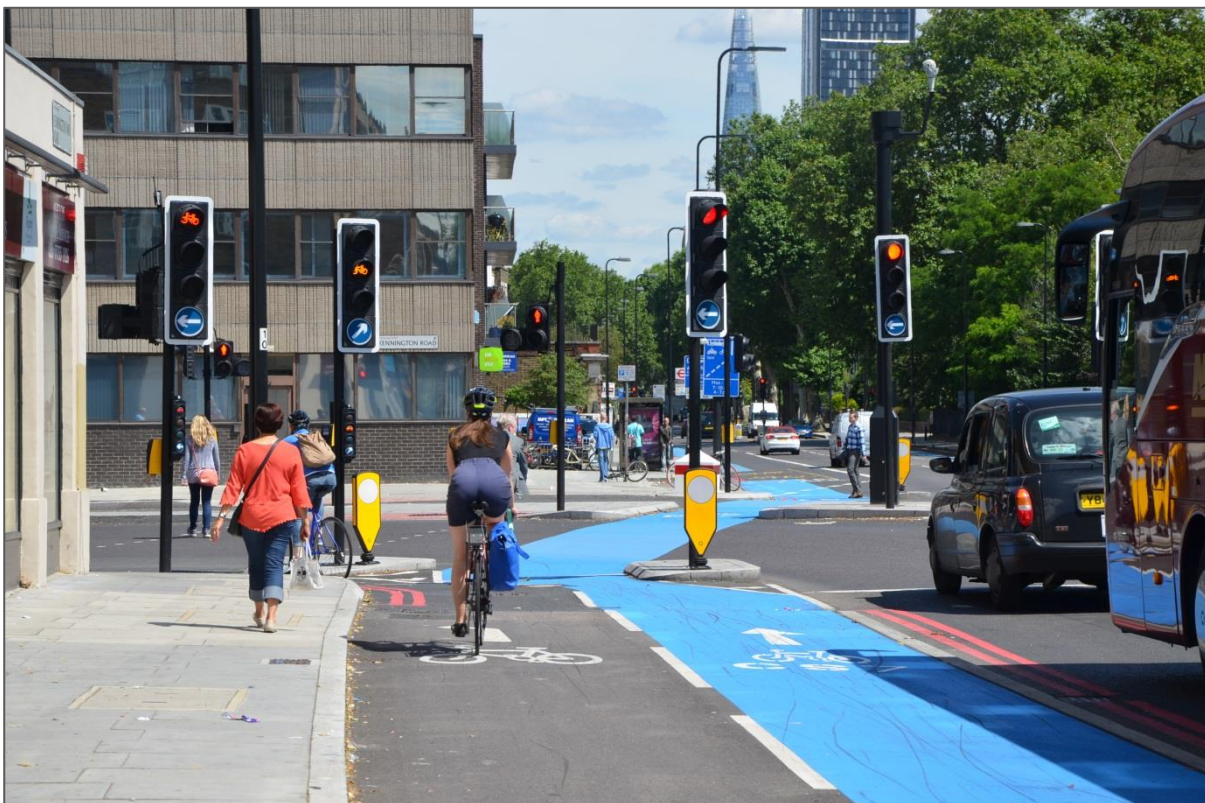
Figure 2: Example of hold the left technique
