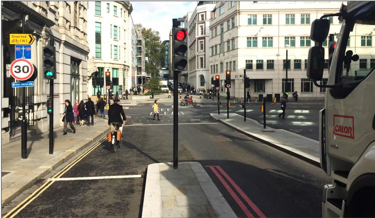
Figure 5: Example of cycle gate technique
