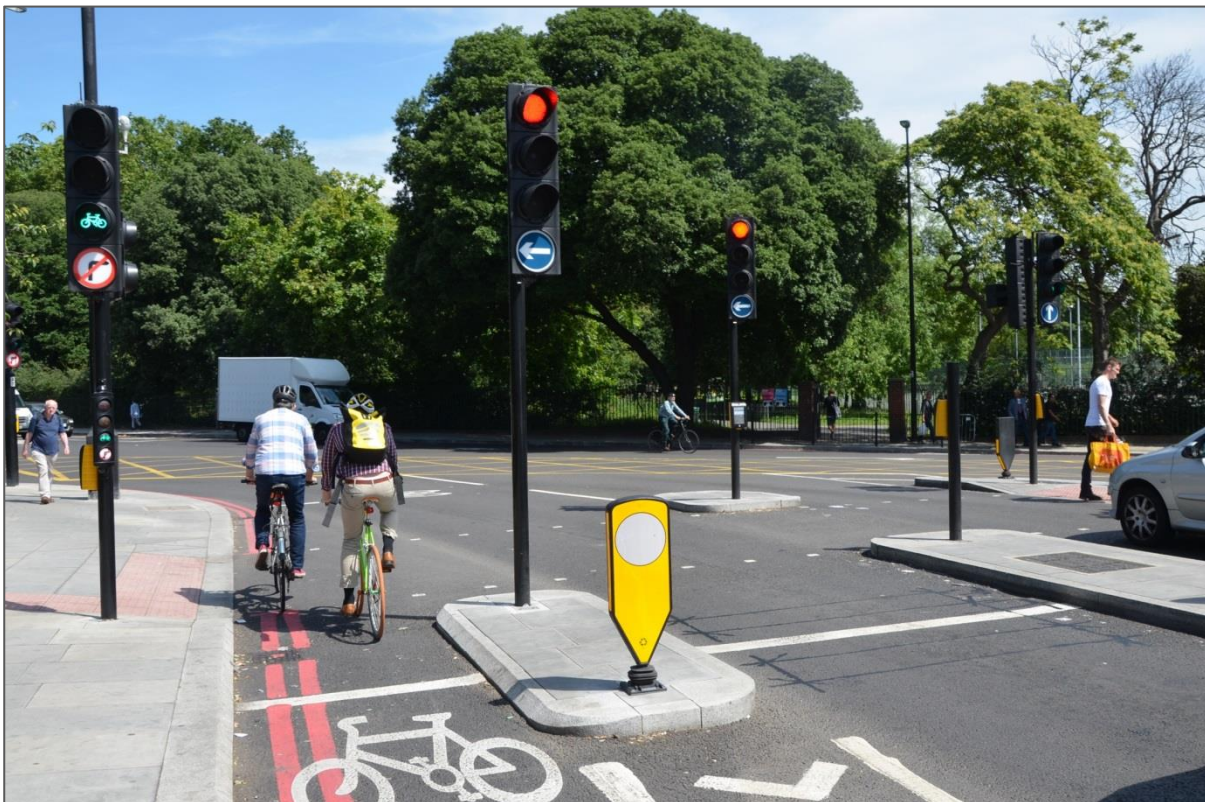
Figure 3: Example of early release technique
