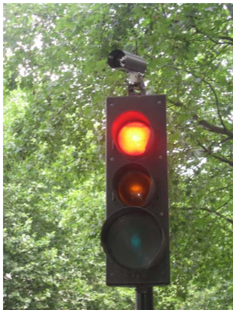
Figure 5.1 A typical semi-permanent automatic number plate recognition camera installation on a traffic signal head.
