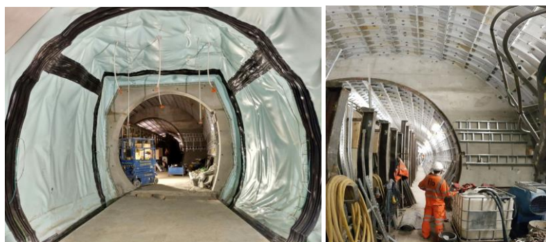
Above –waterproofing of the tunnels and construction of the headwall
