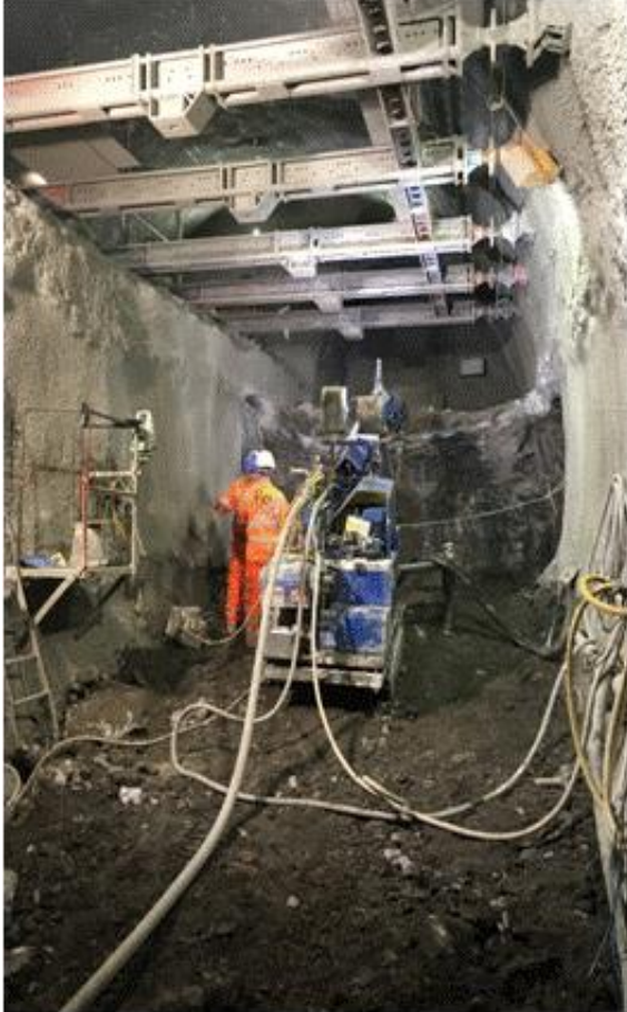
SCL Invert tunnel W/C – 14/11/2016
