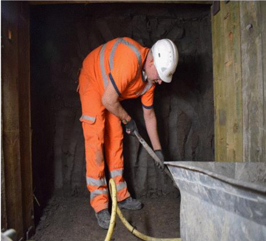
Installation of timber heading December 2016
