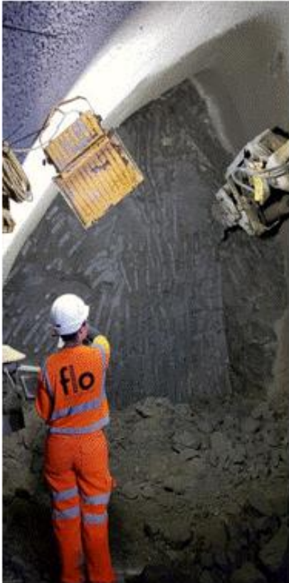
Pilot tunnel W/C – 24/10/2016
