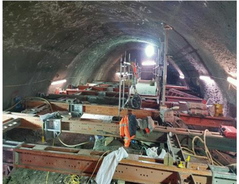
Props installation on over dig tunnel WC 14/11/2016
