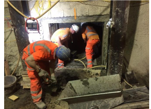
Timber Headings underneath Kennington Loop
