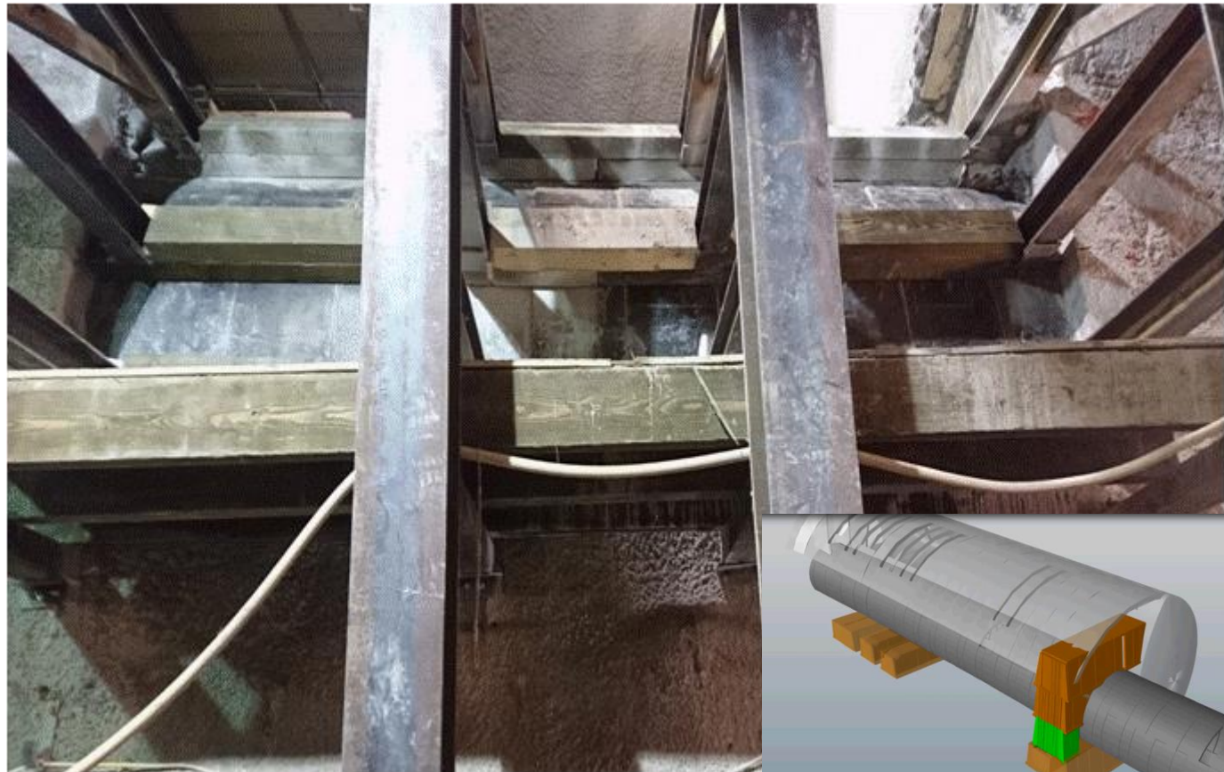
Installation of timber heading WC – 05/12/2016
