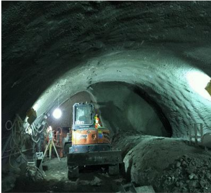
Overdig tunnel with live tunnel right bottom W/ C – 07/11/2016
