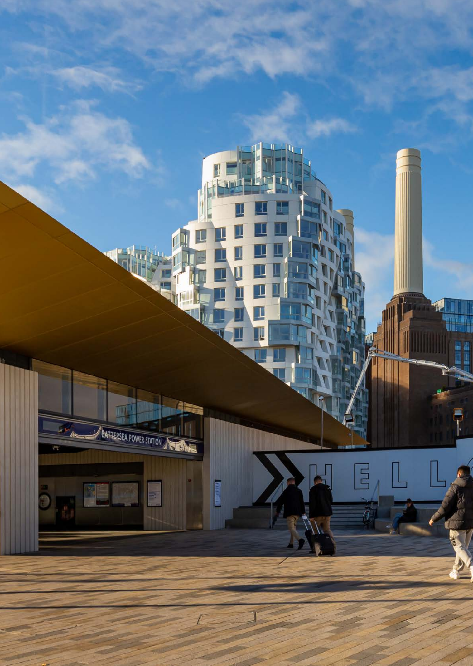
The Northern line now extends to Battersea Power Station
