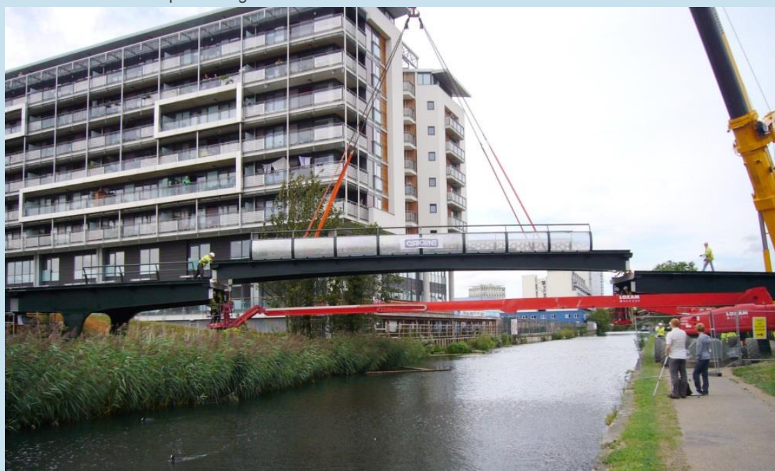
Installation of the Meath Bridge in 2009. © Sustrans
