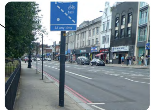
Clutter: redundant posts and columns line footway on west side
