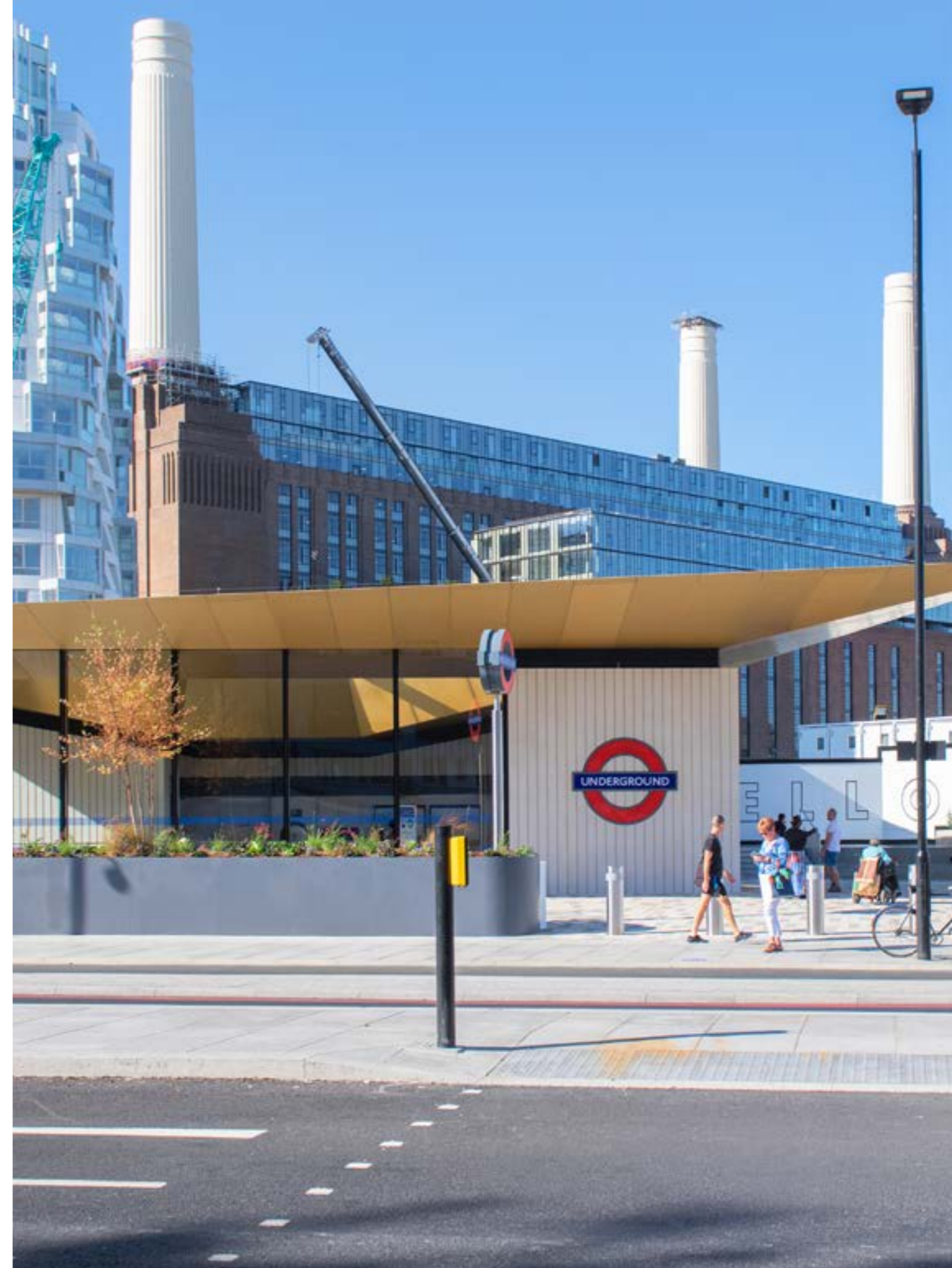
Double the number of trains now serve the new Northern line extension
