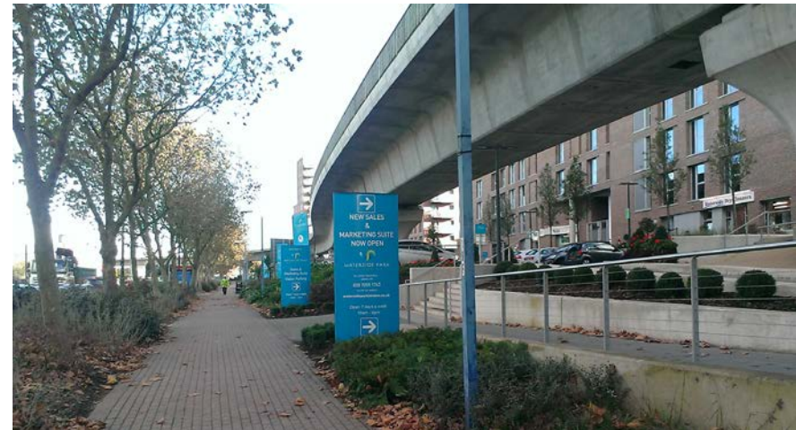
Above from top: DLR viaduct, looking westward from Pontoon Dock Station Landscaping beneath DLR viaduct, Barrier Park East development (North Woolwich Road)
