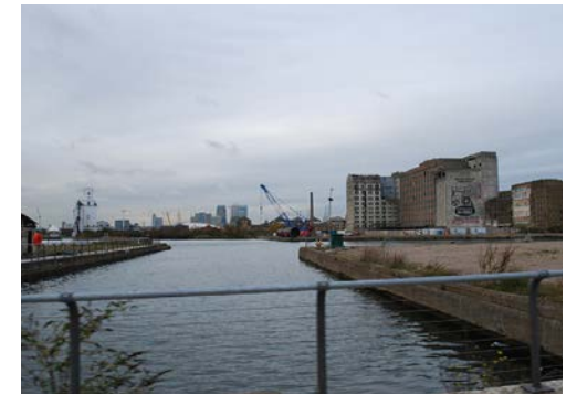
Dock edge treatment E
