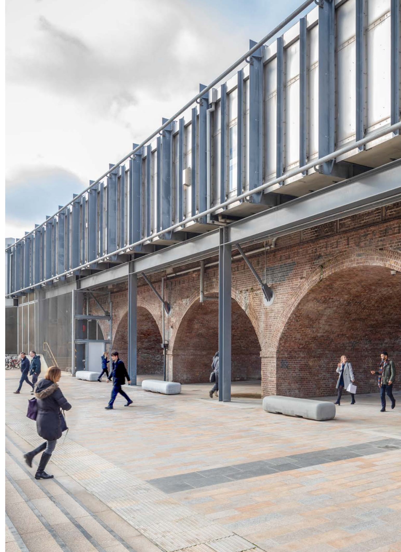
We are creating more retail units in our railway arches
