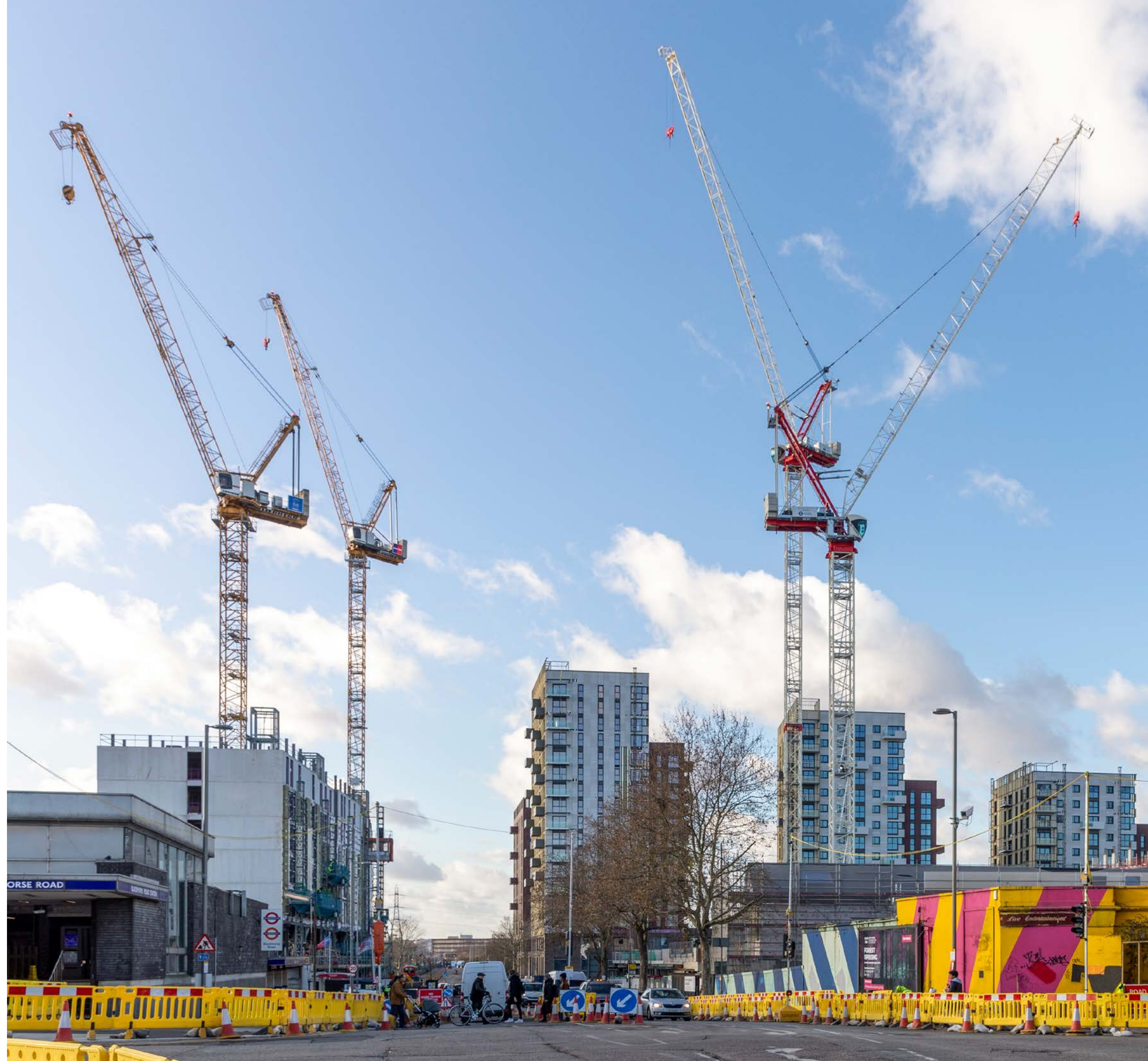
Work continues to improve the area around Blackhorse Road
