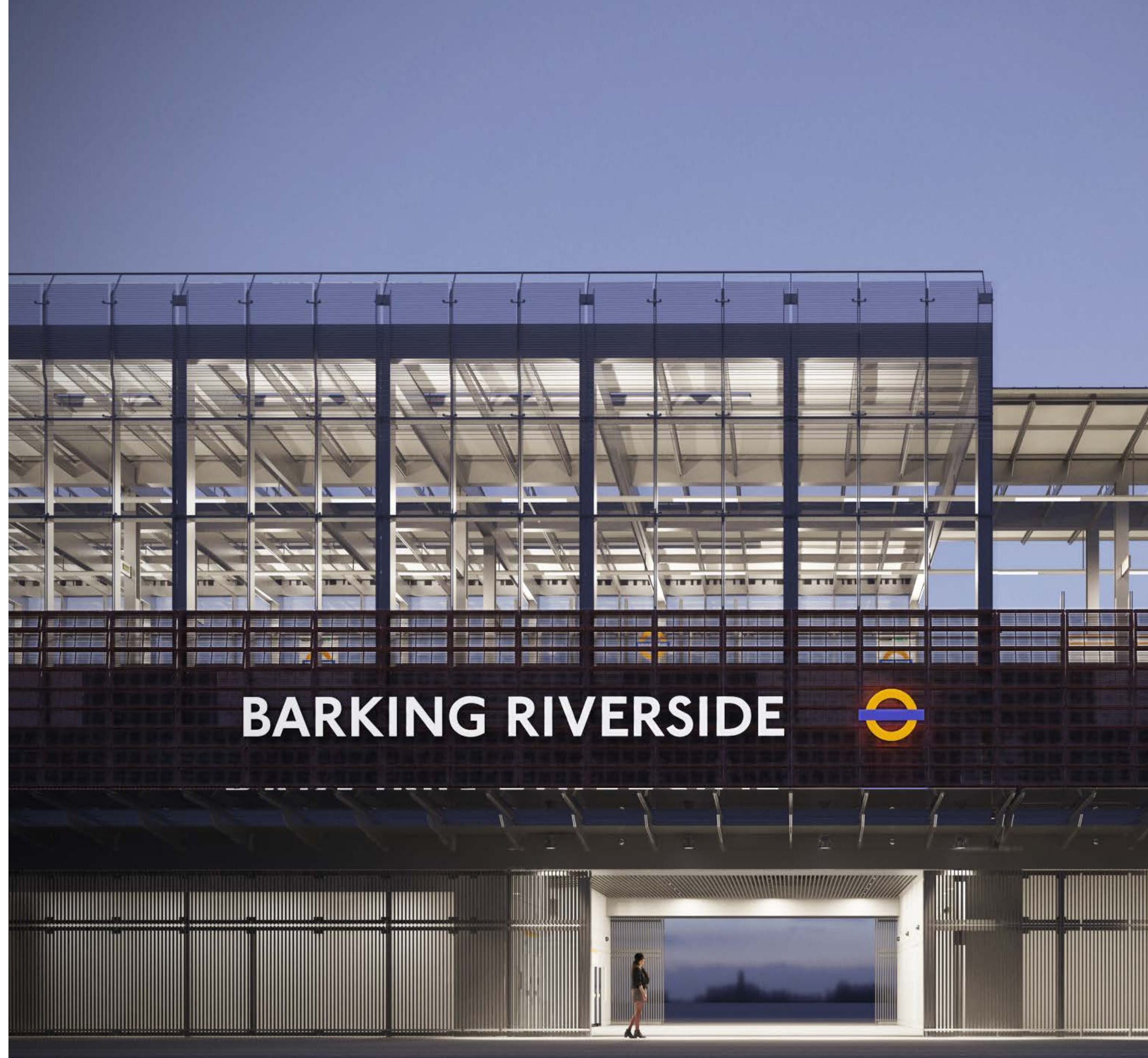
The Barking Riverside Extension will help serve new homes
