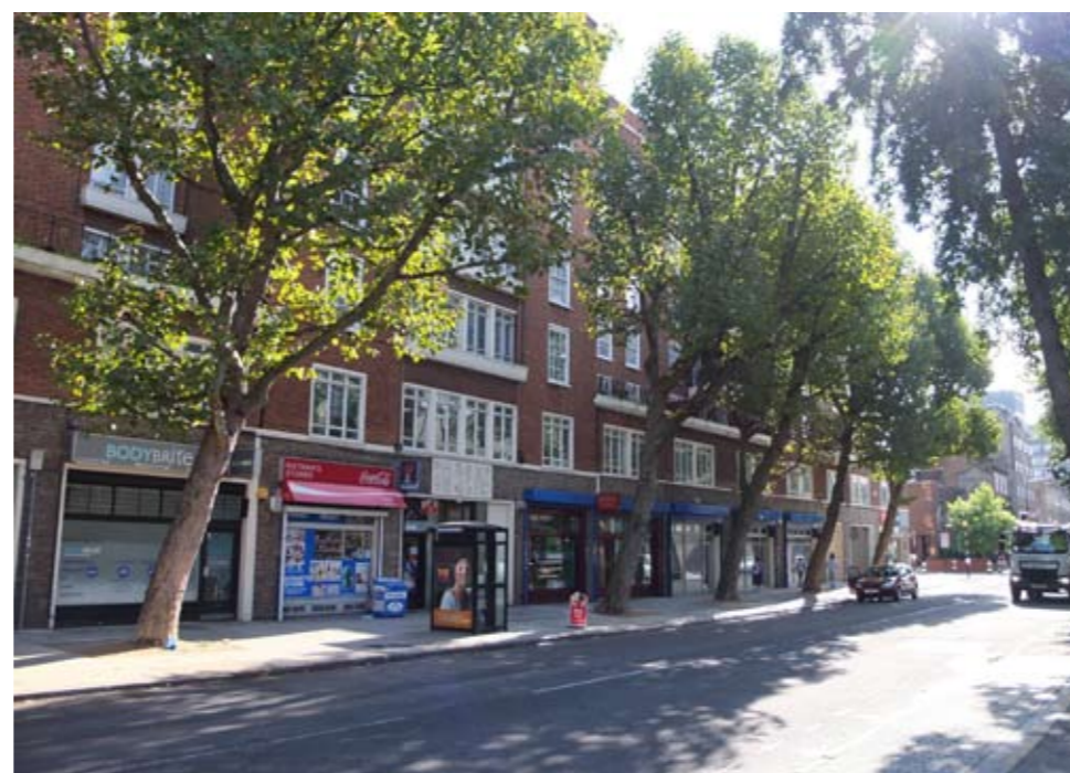
6 Trees make Eversholt Street more attractive. The east side is animated by active frontages.
