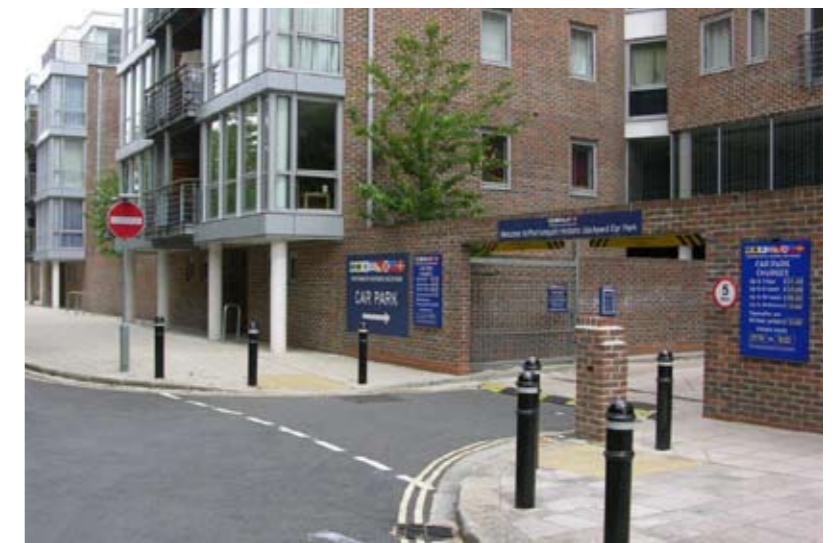
Car park wrapped by block of flats in Portsmouth
