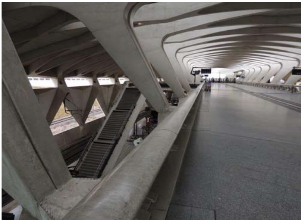
Height change within a walkway is accommodated at Lyon Saint-Exupéry TGV station
