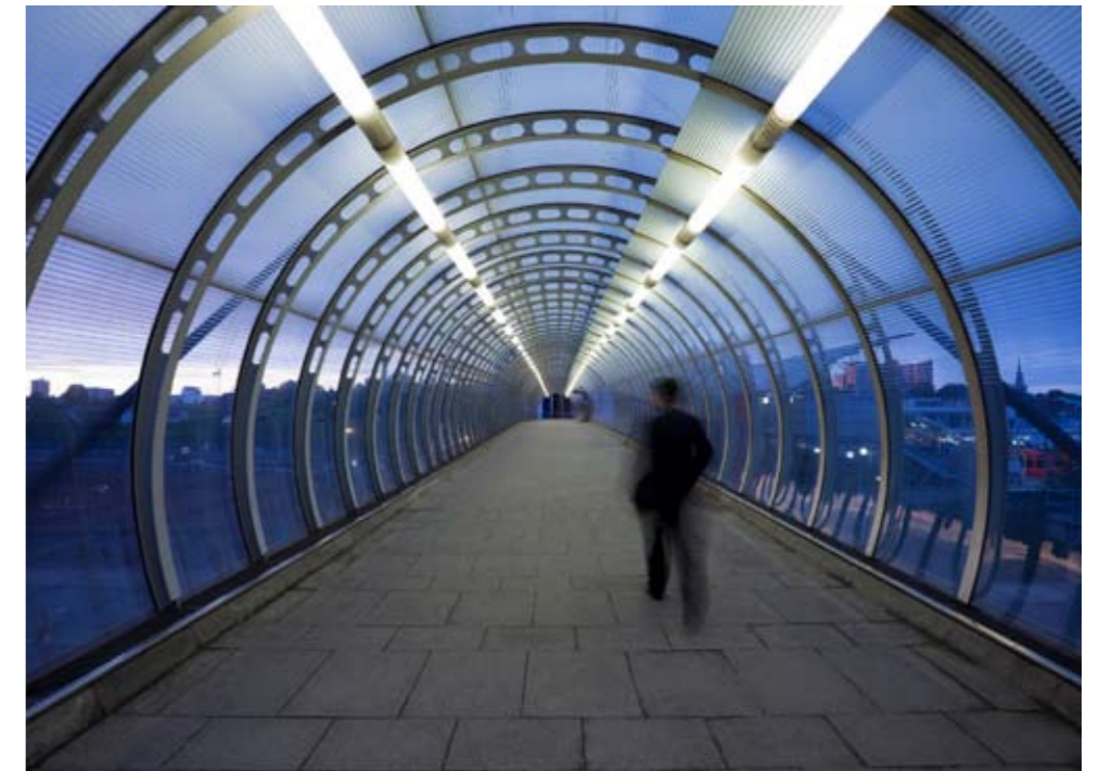
Poplar DLR footbridge crosses the A1261 and the adjacent railway lines. It also allows passengers to access the DLR platforms.
