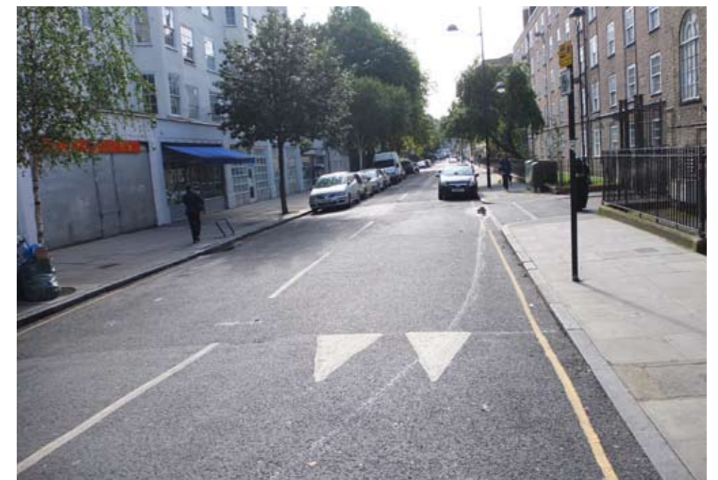
5 Both sides of Phoenix Road are bounded by large blocks of medium-rise flats. Walker House (RH building) is inward-looking, deadening its frontage to Phoenix Road.
