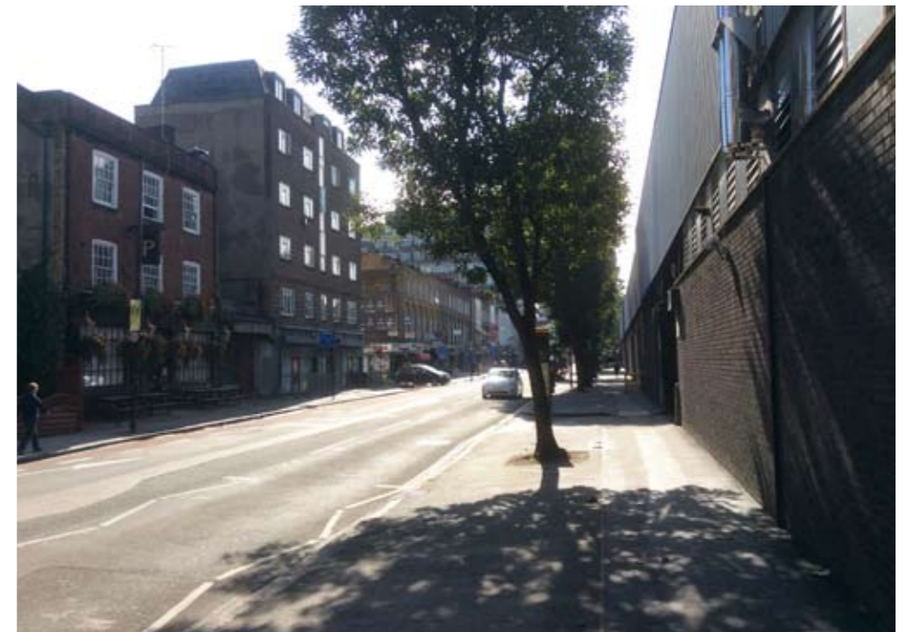
7 The busy frontage along the east side of Eversholt Street provides a welcome contrast to Euston's blank walls.
