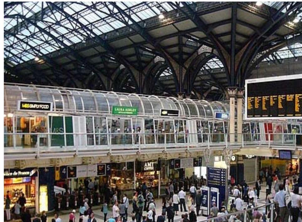
The walkway at Liverpool Street station spans all platforms. It also accommodates shops
