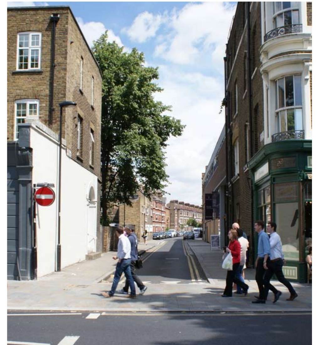
Continuous footway improves pedestrian comfort
