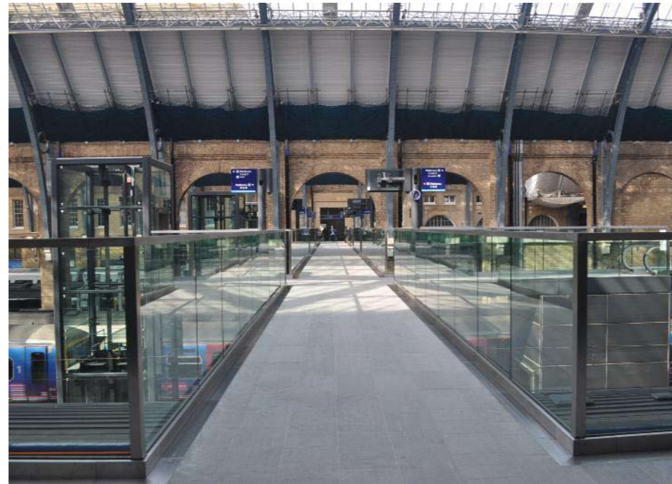
Glass footbridge provides access to platforms at King's Cross
