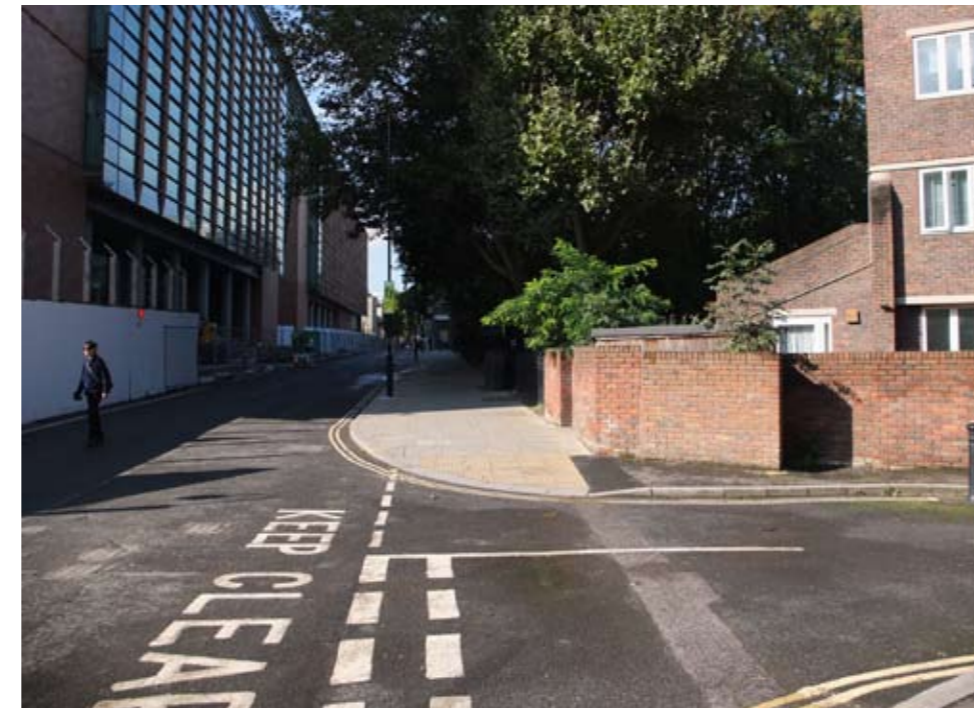
7 Splayed junction layout at Neville Close is not optimised for pedestrian comfort.
