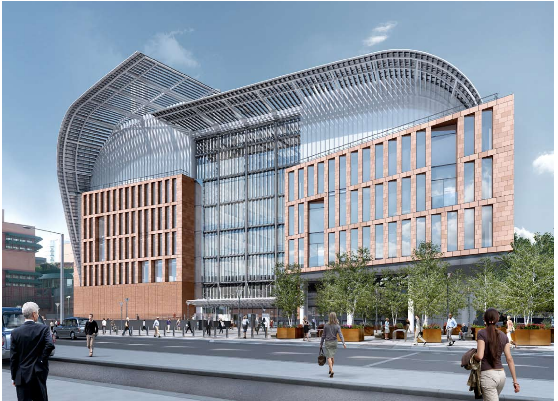
East entrance to Francis Crick Institute (image: HoK)
