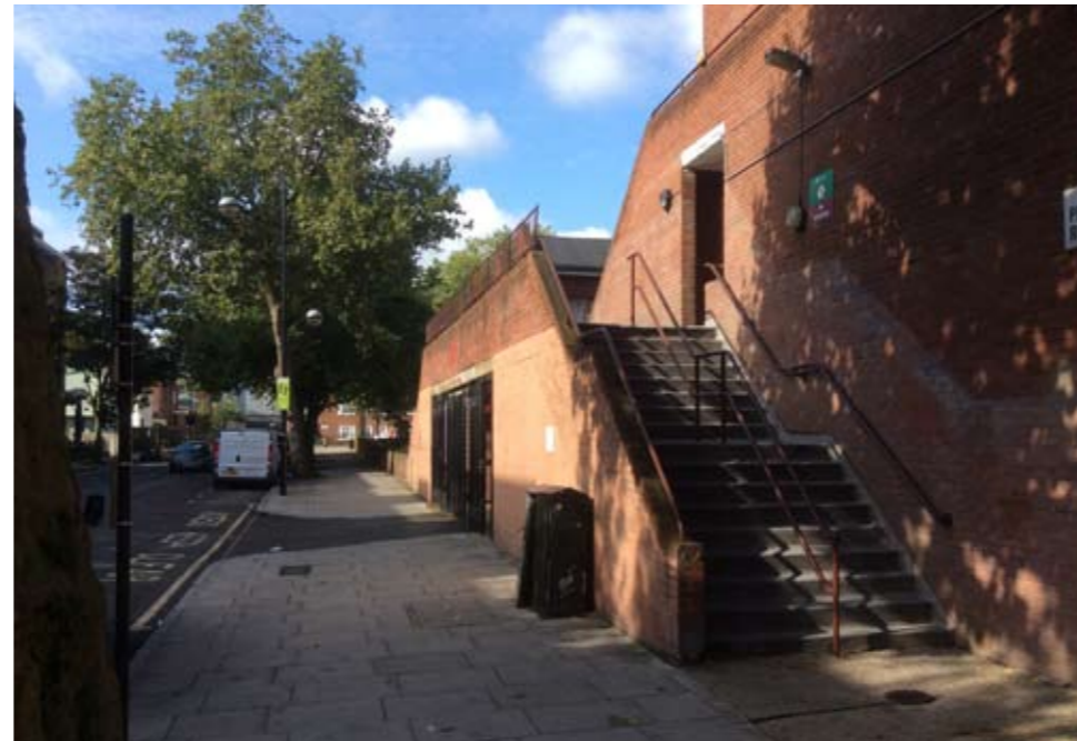
③ 1970s flats have a poor relationship with the street. This section of Phoenix Road is quite incoherent.
