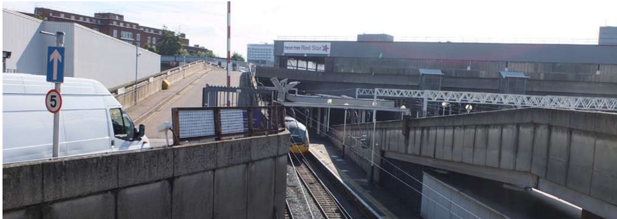
2 Access ramps to Euston's platform and parcel deck are visible from Barnby Street, to the north of the station.
