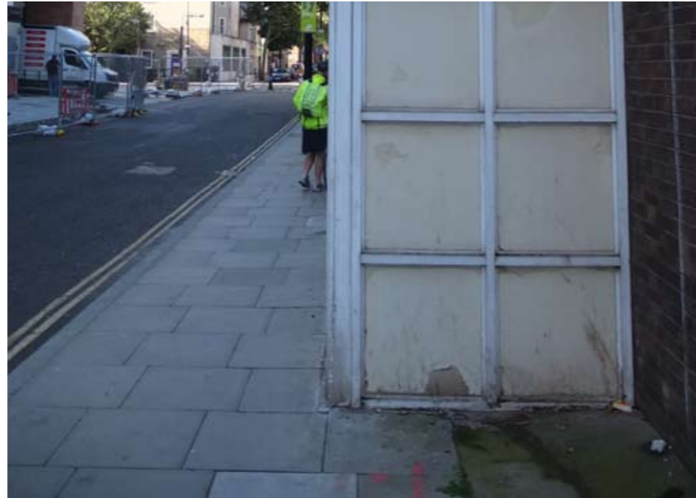
3 This building's stairwell restricts the width of the footway.
