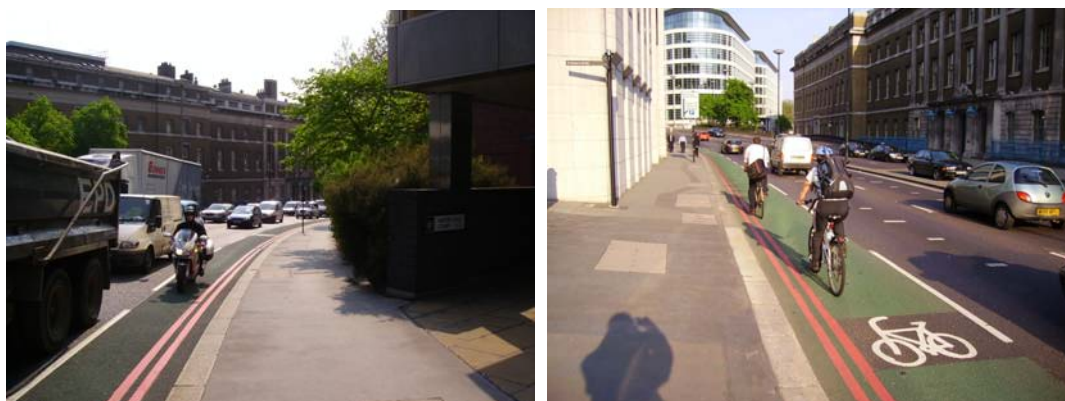
Figure 3.1 - Byward Street cycle lane on approach to Great Tower Street junction
