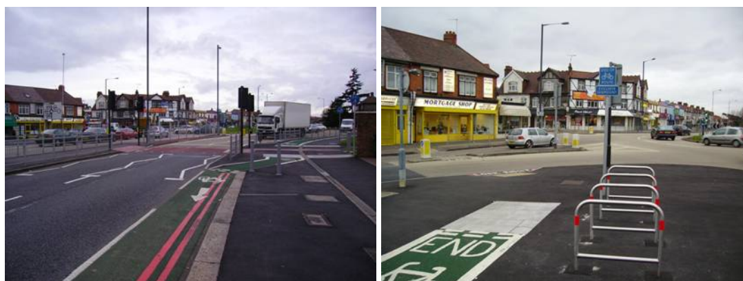
Figure 8.2 - Protected transition from cycle track to cycle lane (left); Cyclist dismount sign next to new cycle parking (right)
