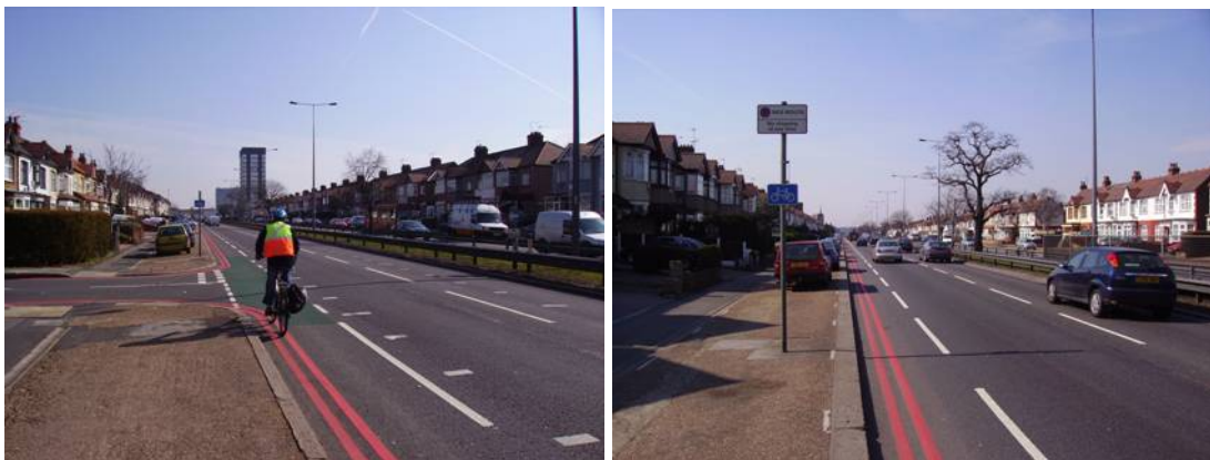
Figure 7.1 - The A12 Eastern Avenue cycle lane
