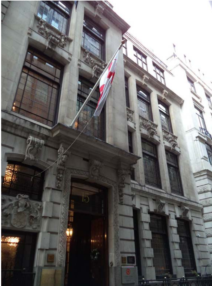
Photo 1: General view of 15 Abchurch Lane
