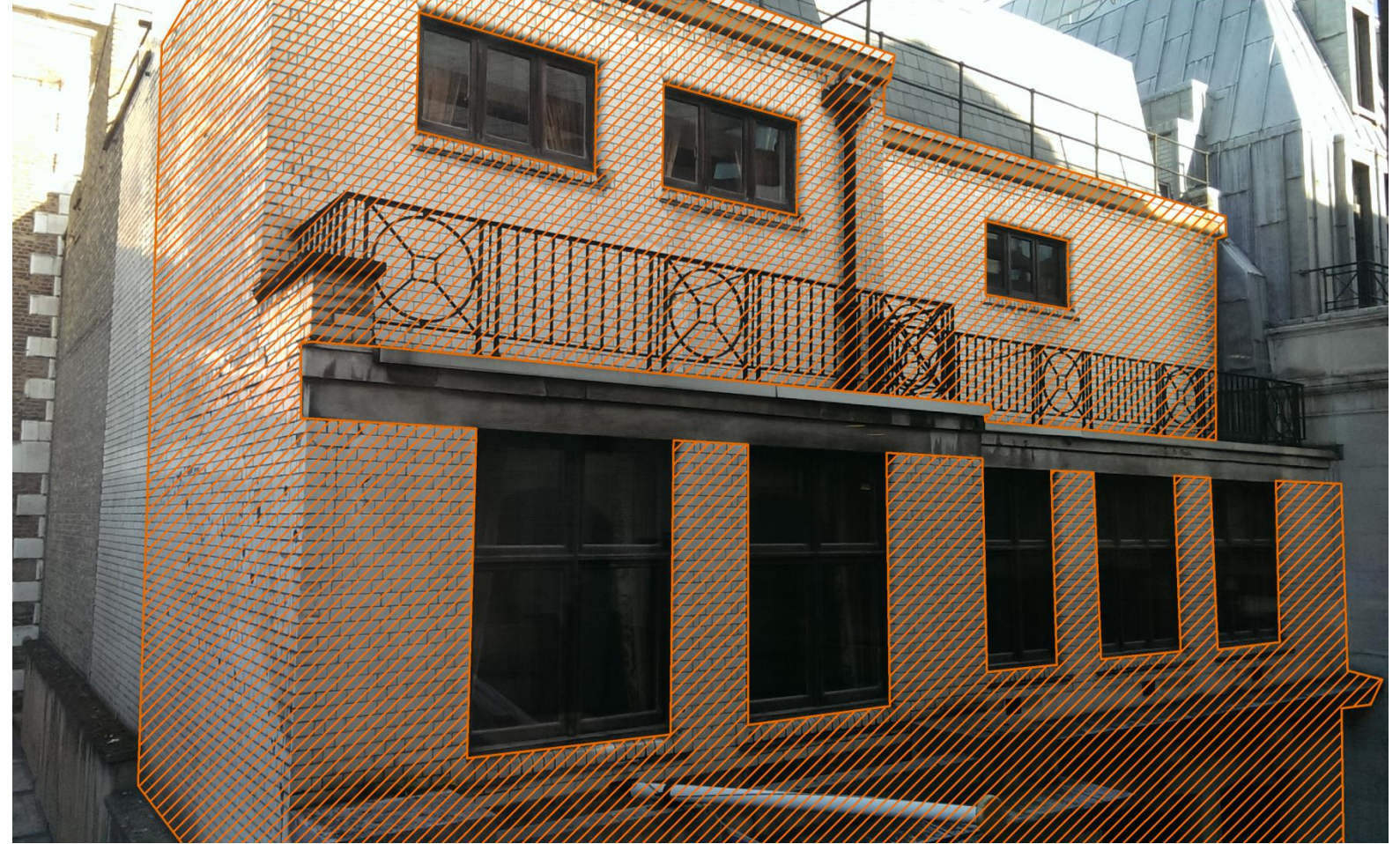
Hatching denotes areas of stone and brickwork which may require protective works following survey
