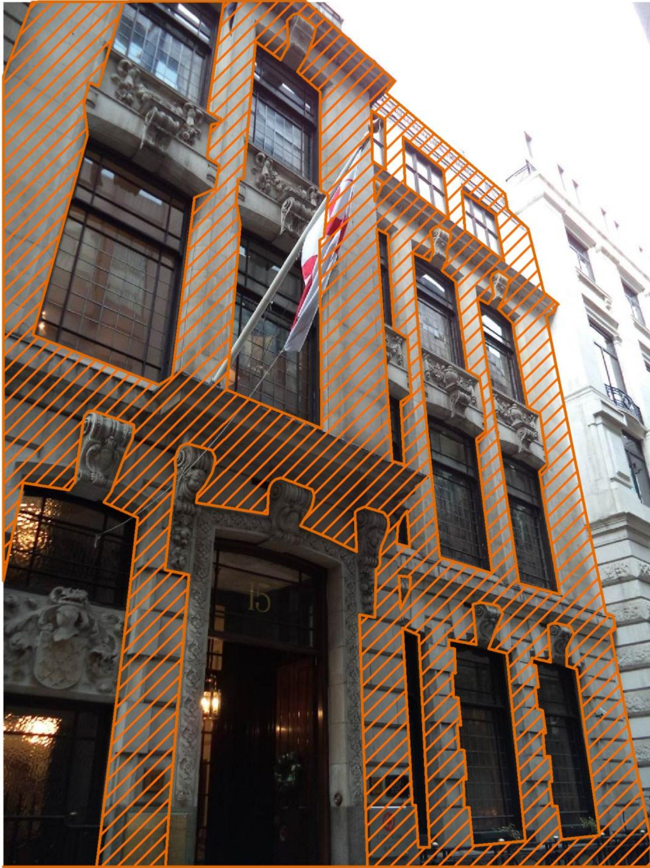
Hatching denotes areas of stone and brickwork which may require protective works following survey
