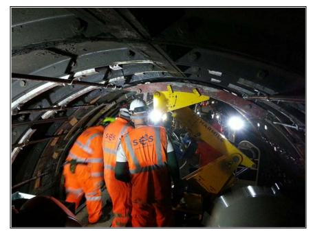
Cutting head being readied to begin removal of crown section of expanded concrete ring.
