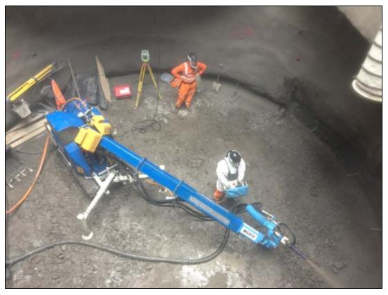
Bond Street concrete lining spray of shaft I
