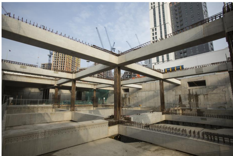
Above – basement level – 1 of the station box
