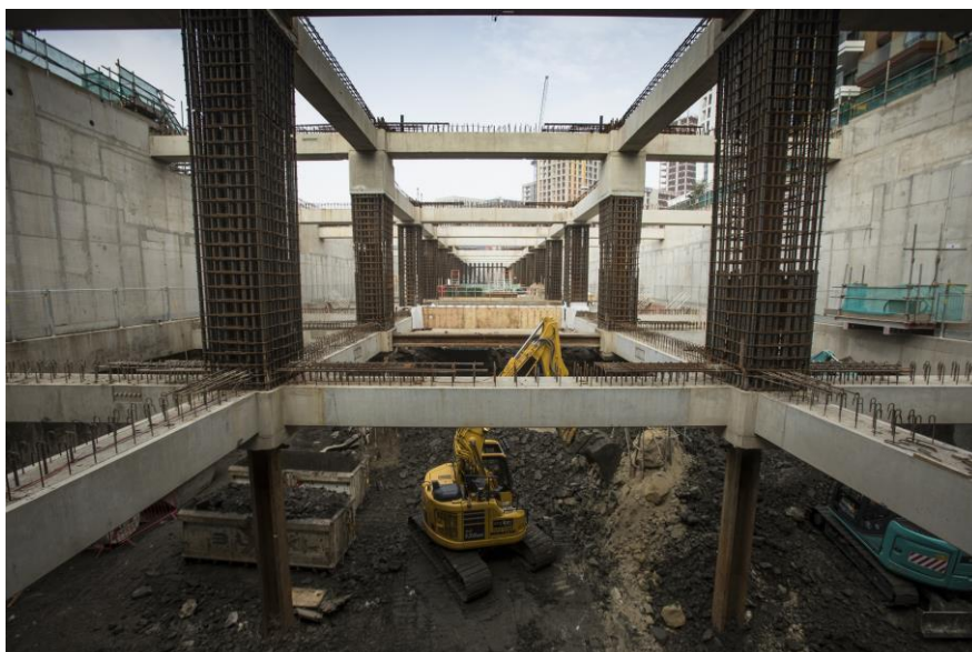
Above – excavation within the station box to basement level -2
