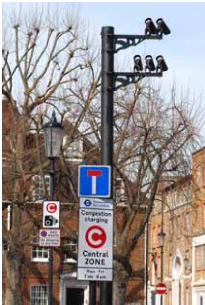
Figure 14.4 Western extension automatic numberplate reading enforcement camera site.
